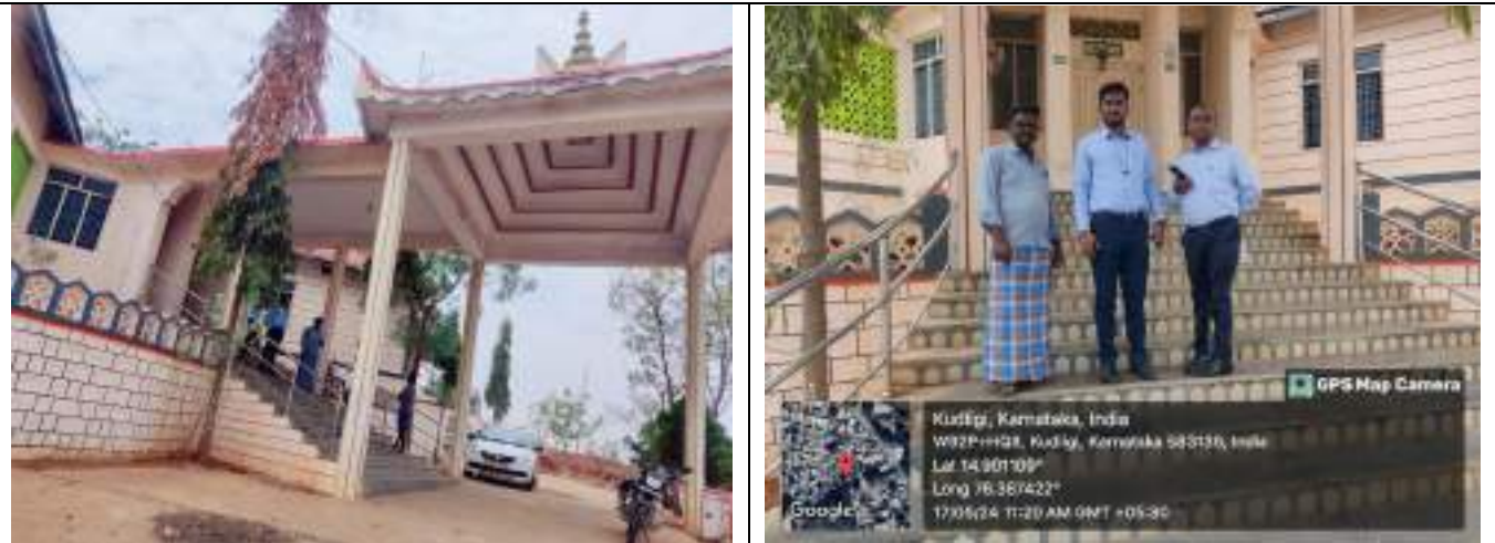
Exterior view of the property
